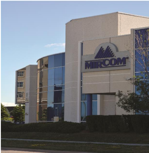
MIRCOM - ENGINEERING & GARDIA OFFICES - SIDE ENTRANCE -
