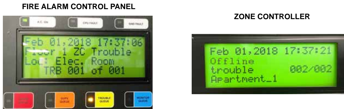
Figure 31 Trouble Condition and Location
