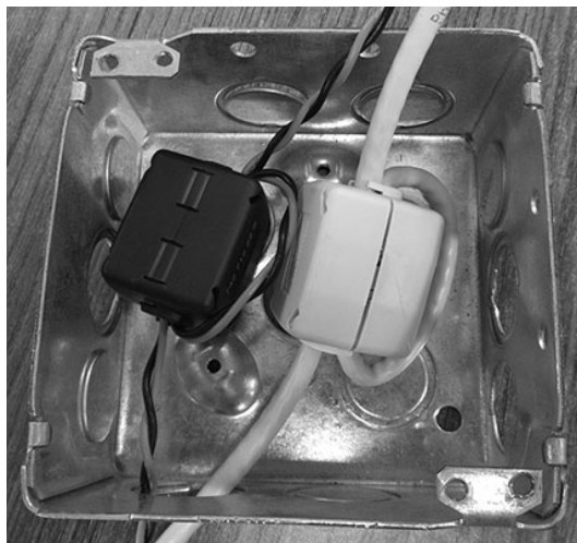
Ferrites installed on the power cable and Ethernet cable in a 4x4" electrical box with a depth of at least 2.7"
